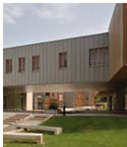
Centre commercial, Gignac
